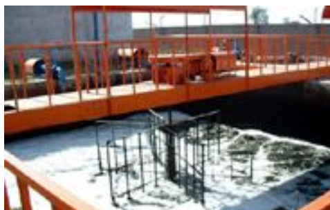
Sprinkling of EM in the equalization tank
